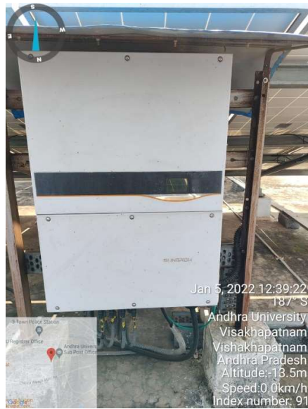
Commerce & Management Inverter 2
