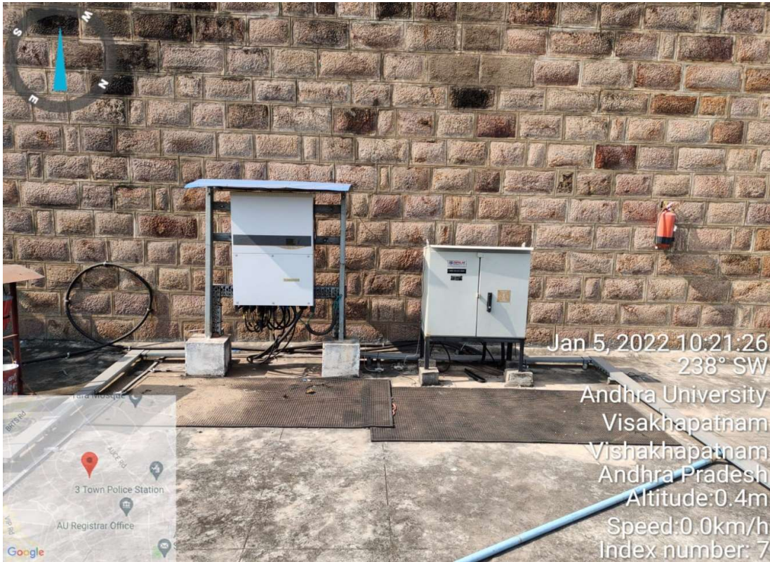
ACDB & 60 Kw Inverter
